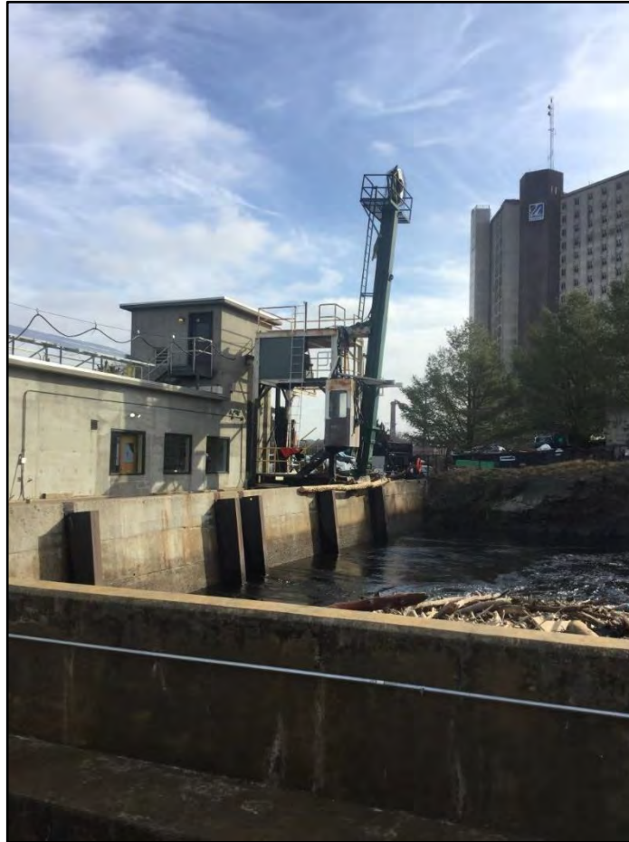
Figure E.7-40. E.L. Field Powerhouse with University of Massachusetts Lowell in the Background.
