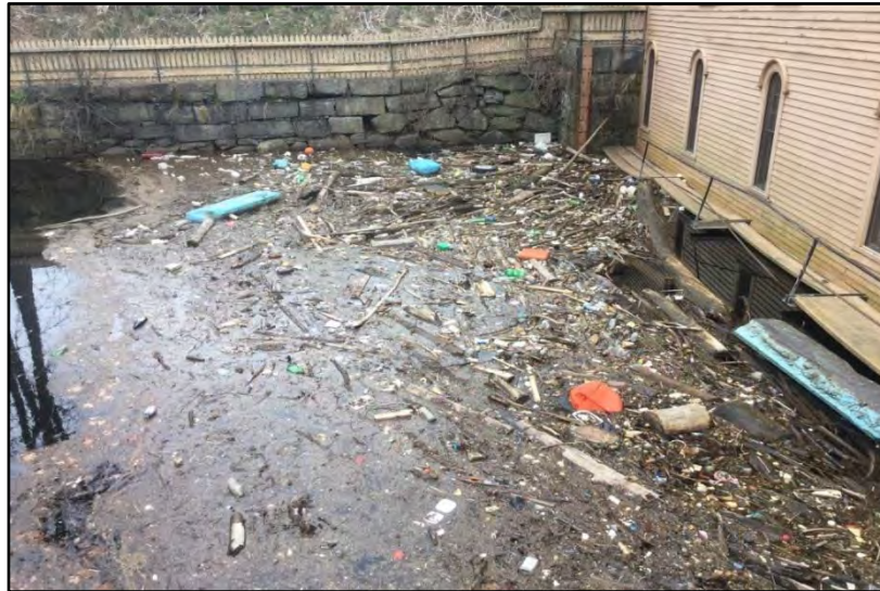
Figure E.7-41. Waterborne trash on the Pawtucket Canal at Guard Lock and Gates Facility.
