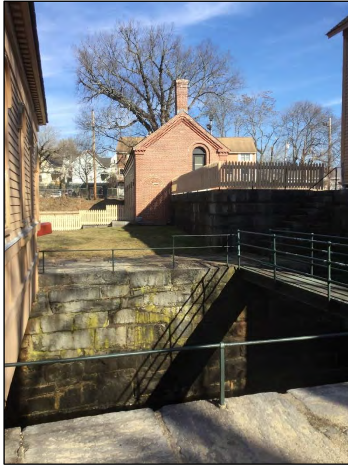
Figure E.7-36. Guard Lock and Gates Facility.
