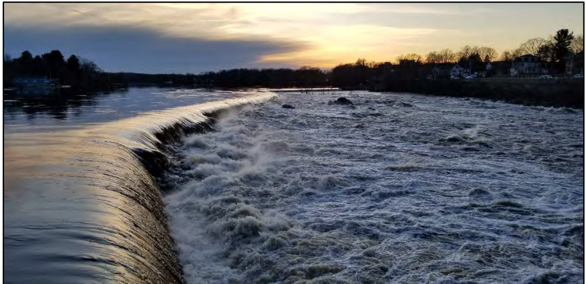
Figure E.7-39. Westerly View of Pawtucket Dam from the Pawtucket Gatehouse
